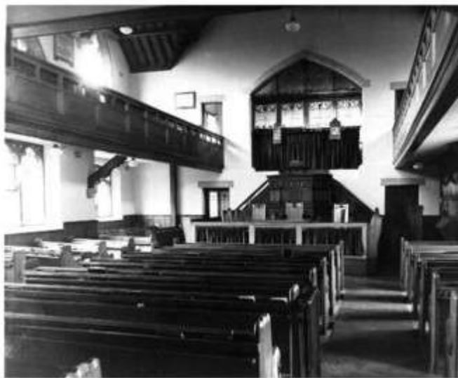
New building Circa 1962. Click on Interior image to enlarge.
